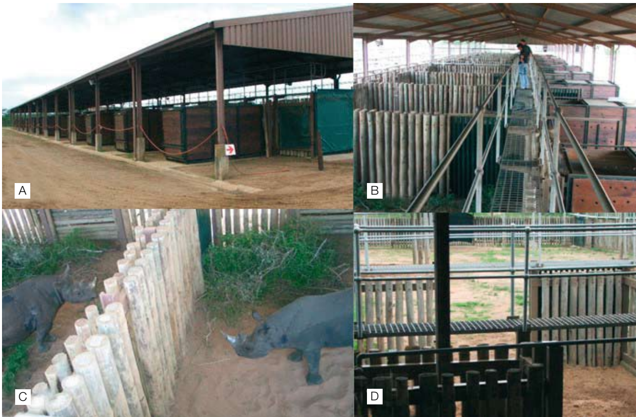
Figure 33: Photos of EKZ's Centenary Game Capture Centre in Hluhluwe-iMfolozi Park. (A) View of outside of rhino bomas showing transport crates attached to boma pens. Note roof to keep rhinos dry and to give shade from the sun. (B) View from an observation gangway at EKZ's Centenary Game Capture Centre. Adjoining wooden transport crates reinforced with angle iron are on the right. (C) Two black rhinos in adjacent pens at EKZ's Centenary Game Capture Centre. Note fresh cut browse which is provided twice daily in addition to lucerne and cubes. Horn transmitters have already been fitted to these animals. (D) Larger white rhino boma connected to smaller inside pens. The incidence of hunger-striking in wild-caught subadult (but not adult) white rhino can be reduced by initially introducing subadult white rhino into a larger boma containing one or more experienced white rhino subadults that are used to feeding in the boma. (Photo credits: Richard Emslie).
