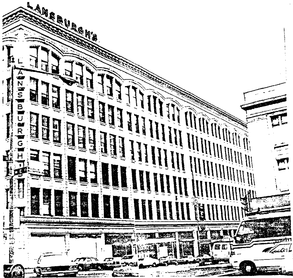
Oblique View of West Facade (Eighth Street)
