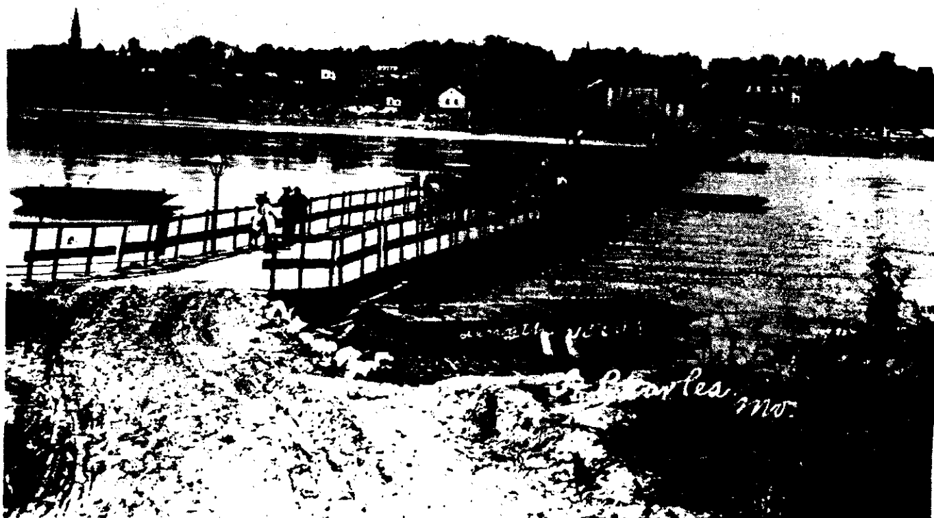
COPY OF 1891 PHOTOGRAPH OF ENOCH'S PONTOON BRIDGE, VIEW TO WEST TOWARDS ST. CHARLES (PHOTOGRAPHER UNKNOWN)
