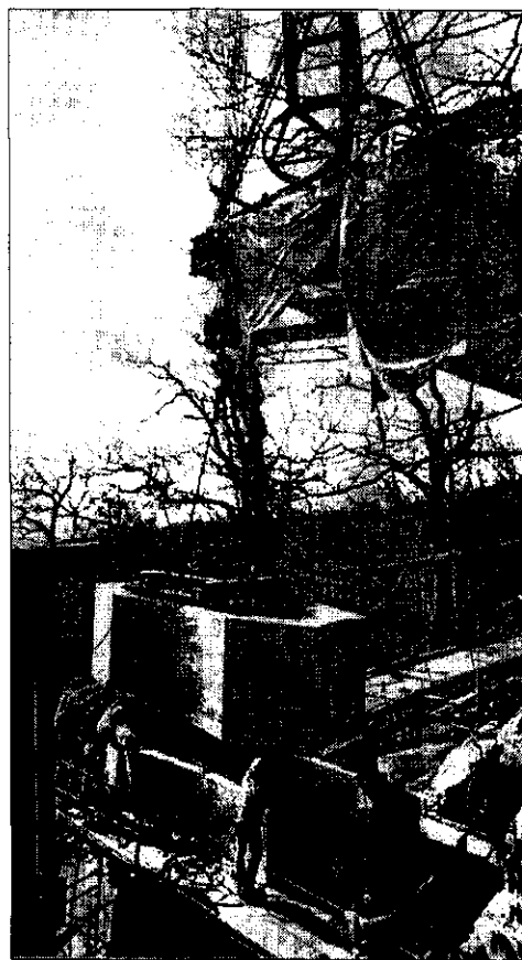
Figure 18 Precast box pier segments were lowered over the end of the completed cantilever with the stiffleg. The workmen are ready to block the segment and apply the epoxy. (Muller and Barker, "Design and Construction," 12)
