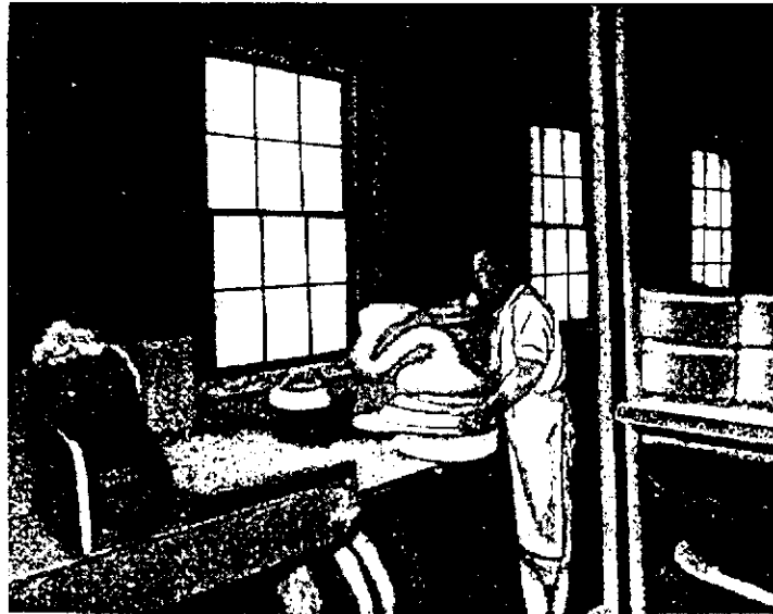
Figure 10. Syphon jet being assembled (Maddock 1910).
