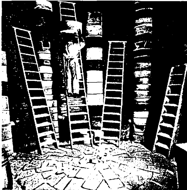
Figure 15. Placing kiln (Maddock 1910).
