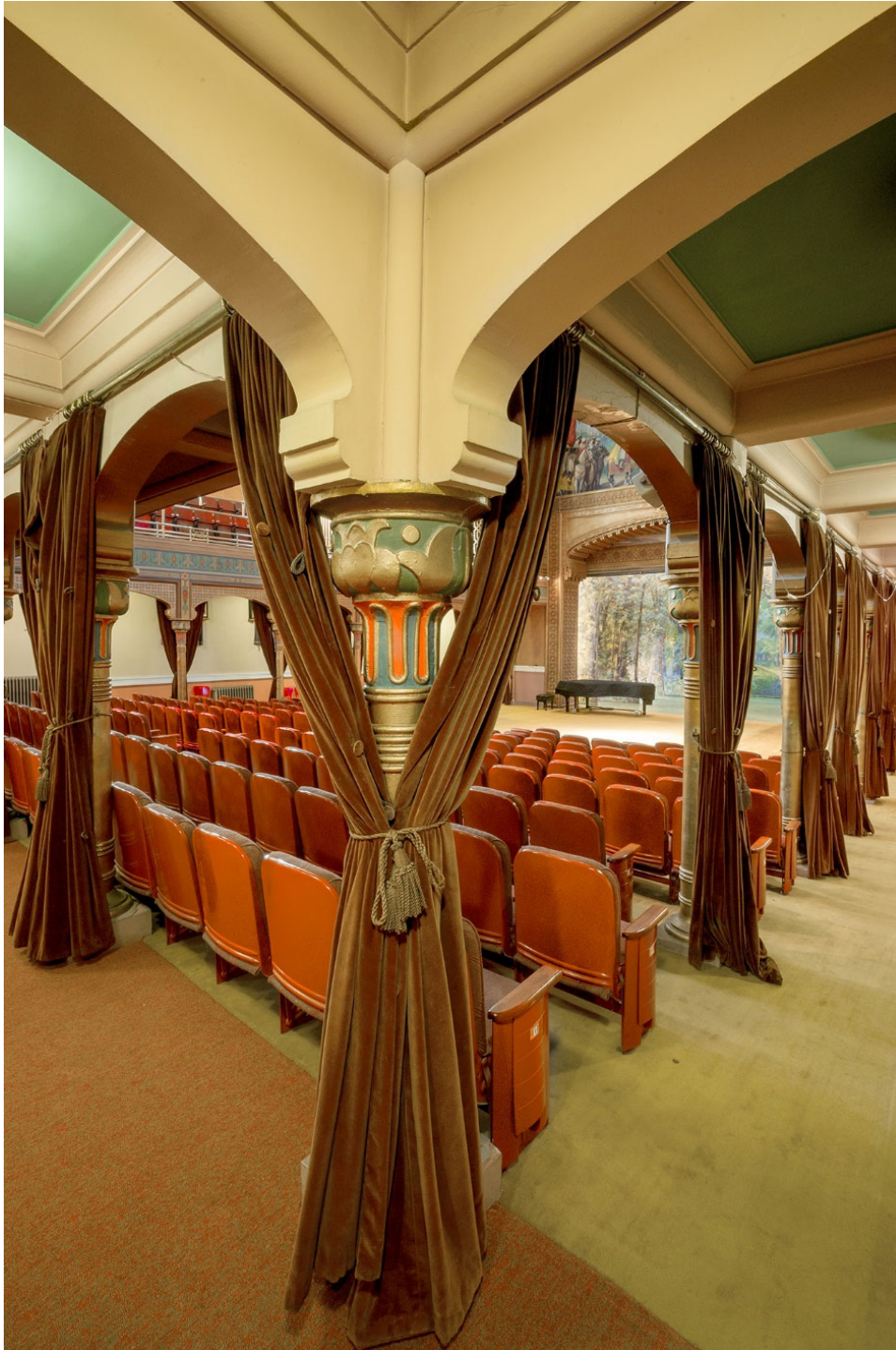
Figure 20. Auditorium showing typical column detail, ceiling coping and drapery; view to southwest.
