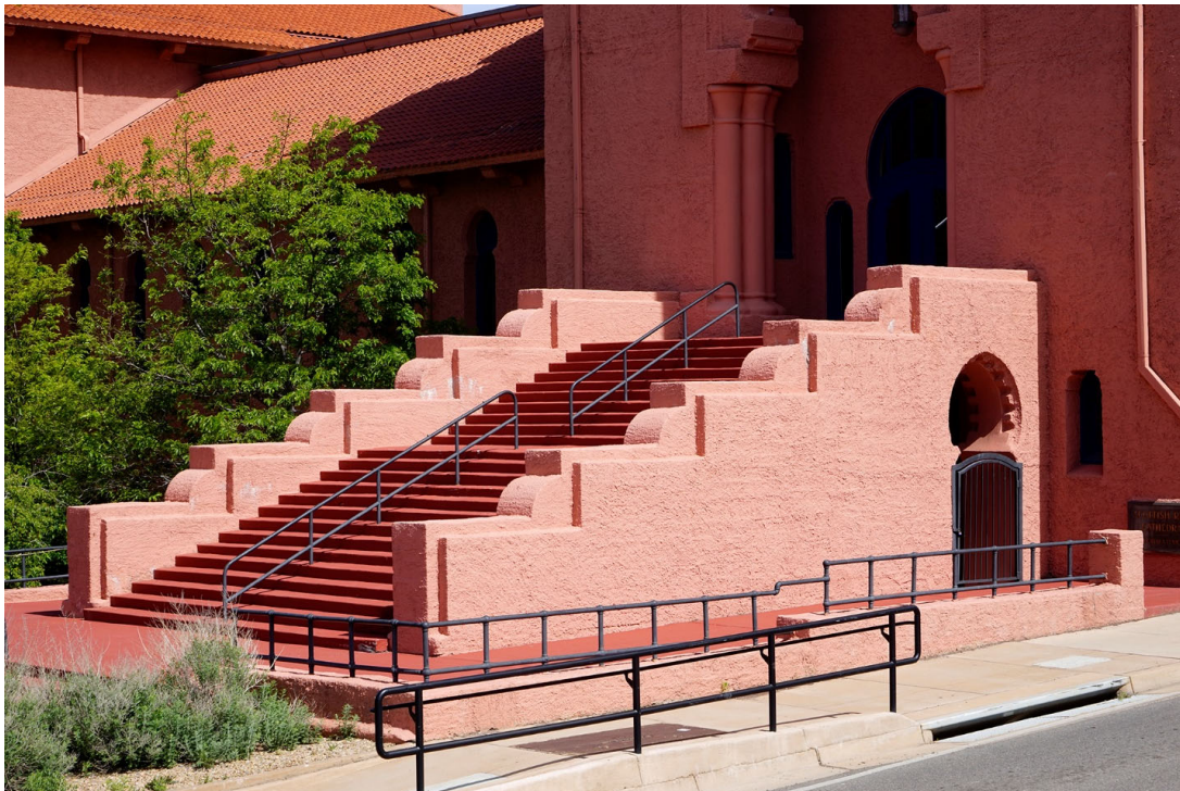
Figure 8. Detail, stairs to main entry on south elevation; view to northwest.
