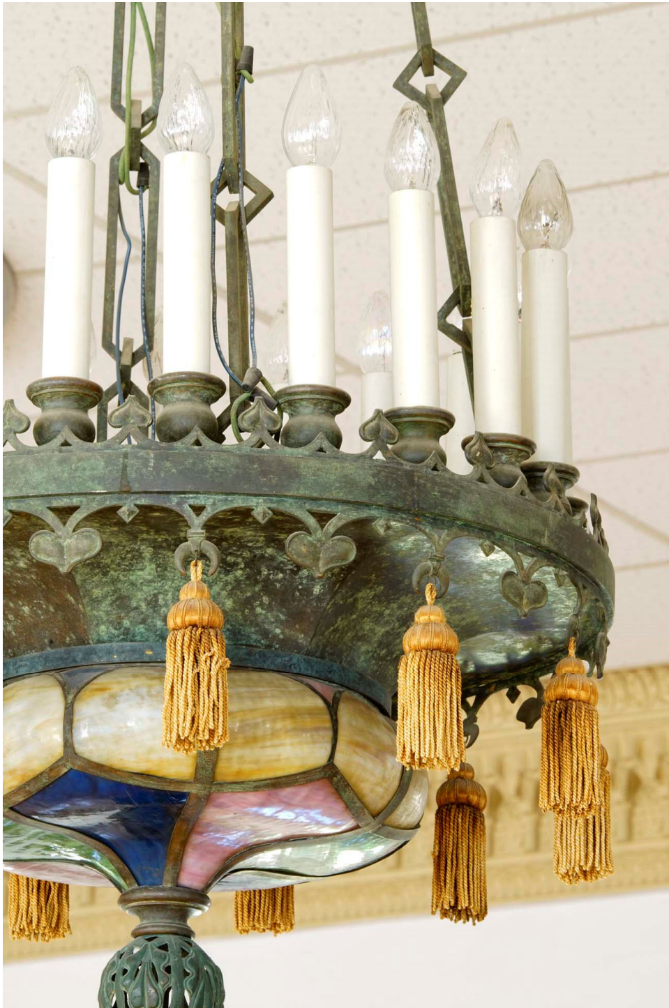
Figure 34. Dining room detail, pendant electric fixture; view to southwest.
