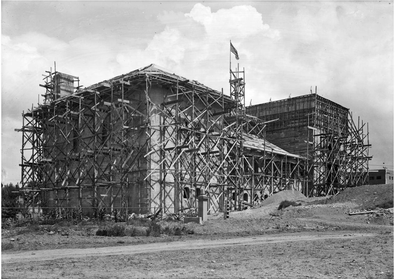
Figure 3. Scottish Rite Temple under construction, 1912.
