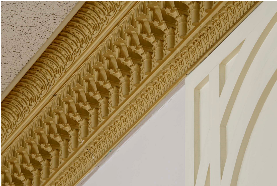
Figure 33. Dining room detail of cove molding on east wall (typical); view to northeast.
