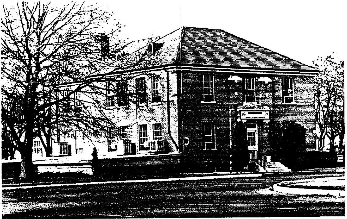
Illustration 2 View of the east and south sides of Building 1. The headquarters building, a two-story brick structure with red clay tile hip roofs, is one of the most architecturally distinctive buildings on the installation. The use of permanent masonry construction for key buildings in the administration area is a characteristic feature of ammunition supply depots constructed before the spring of 1942, when masonry materials became in short supply. (Source: Field inventory photograph, 1984, Barbara Hightower, Building Technology, Inc.)
