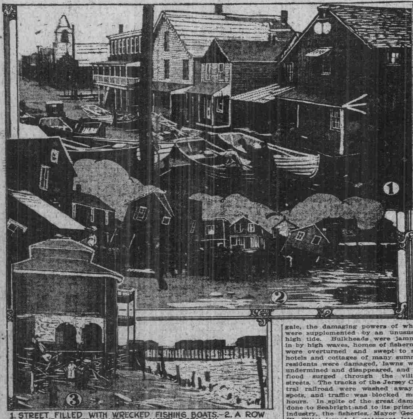
Sea Bright, N. J., Dec. 29.—Ten lives were lost by the foundering of two barges at sea off Barnegat, and property estimated about $750,000 was destroyed in the storm that whipped the New Jersey coast from Sandy Hook to Atlantic City. Seabright, located on a narrow strip of sand between the ocean and the Shrewsbury river, caught the full fury of the sea.
