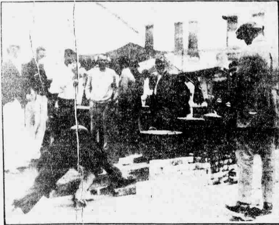
(By Pacific & Atlantic Photos, Inc.—A. T. & T. transmission) Building brick fireplace to feed quake refugees
