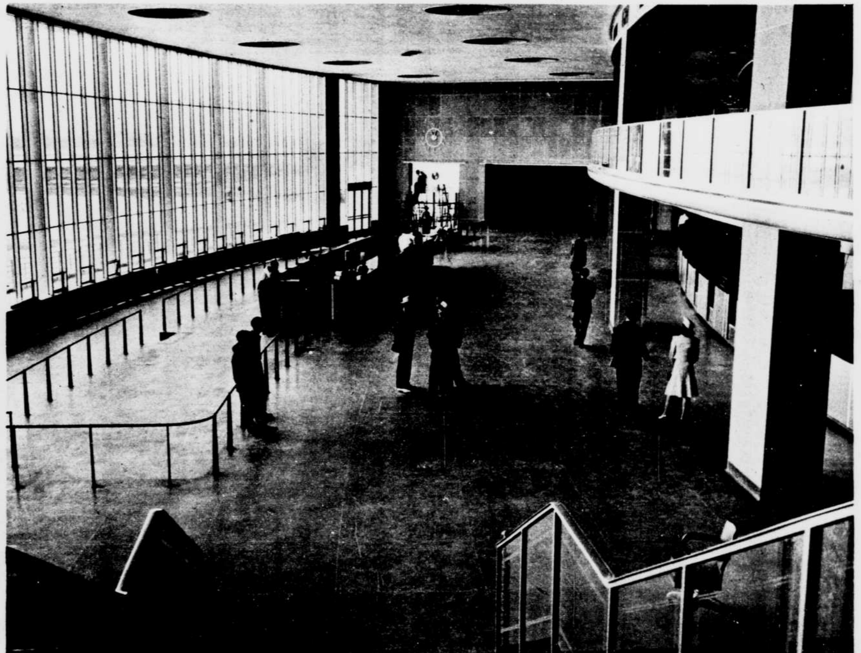
The spacious main waiting room, with its glass-paneled front, looks out on the great pattern of concrete runways that lead the eye to the river and Washington beyond. Here, under the balcony, are the ticket booths, with telegraph stations in the center.
