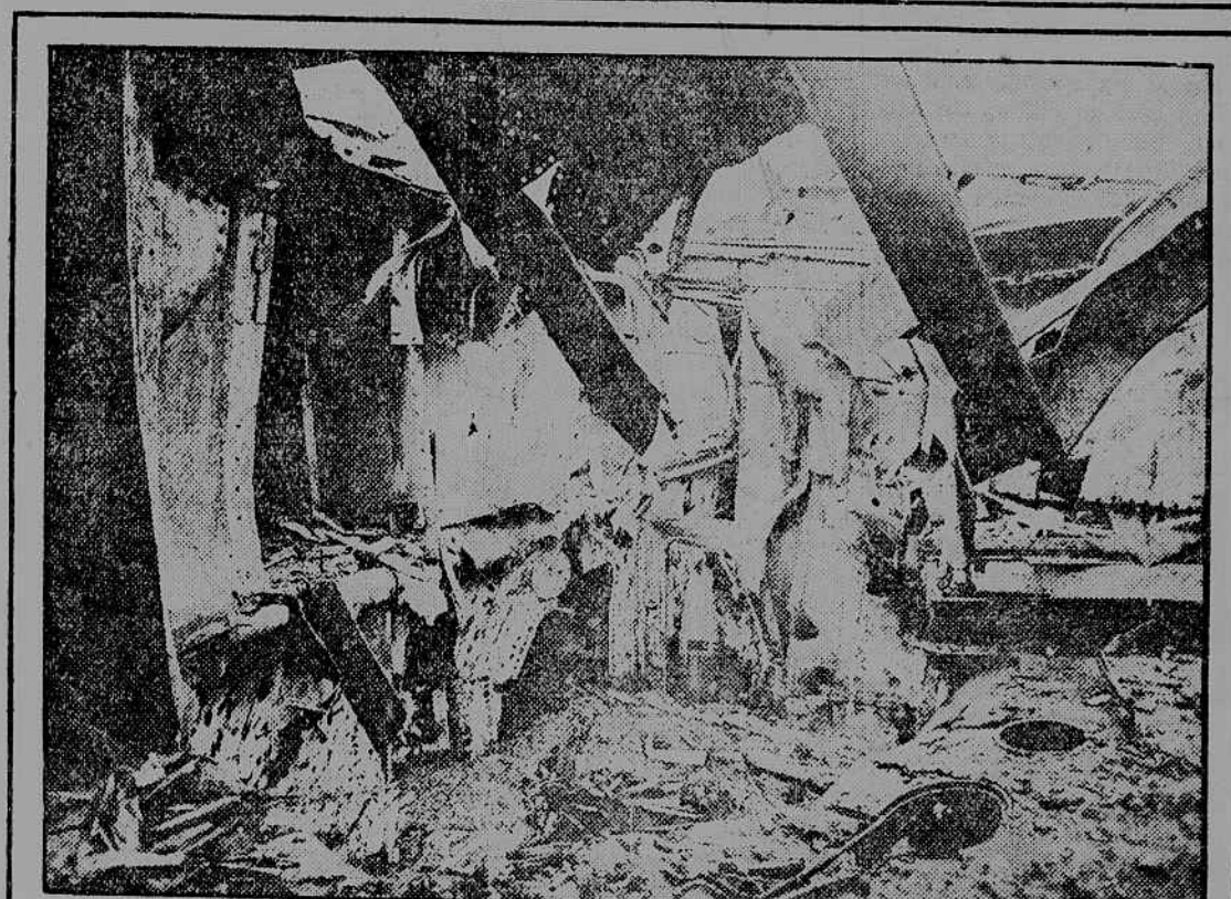
THE bomb was placed aft of the forward 8-inch turret at the point indicated by the arrow AT the left is a view of the vessel amidships, the first deck being blown away AT THE right is a view of the second deck looking forward, the X showing where the bomb exploded THE picture at the lower left hand shows the third deck and the ammunition hoist. Had the ship been in commission the magazine probably would have been exploded AT the lower right hand is shown the destruction wrought on the fourth deck
