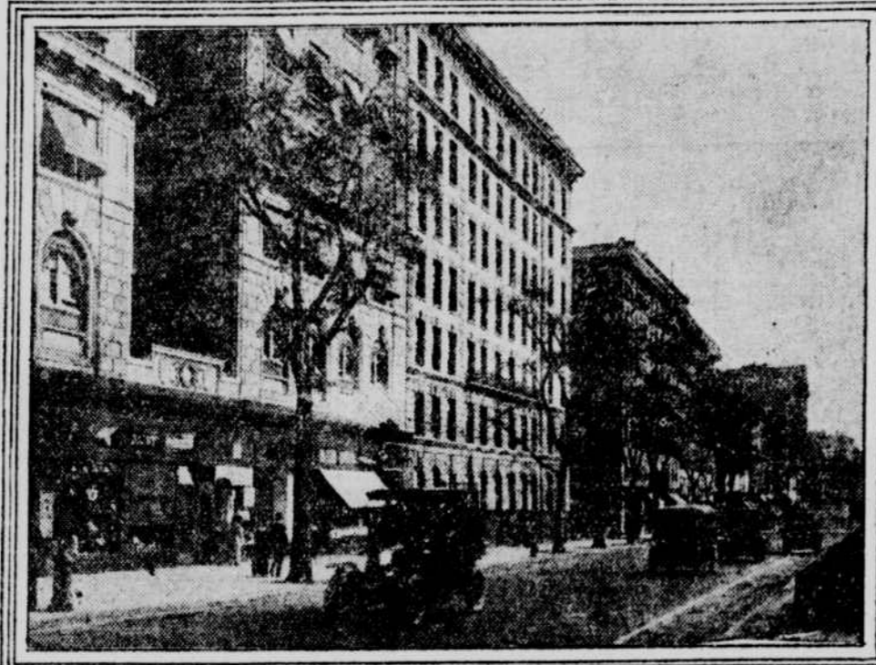
This centre, at 96th street and Broadway, has enjoyed subway facilities since 1904
