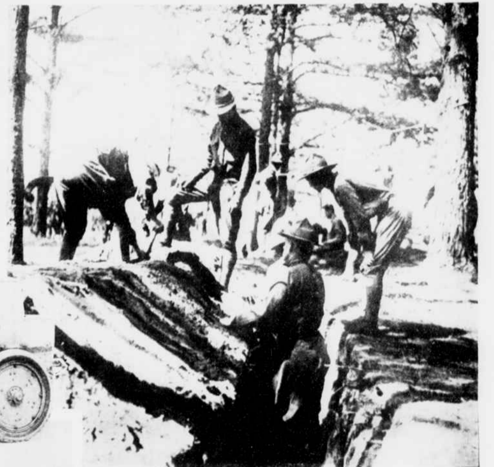
Not spectacular but useful—trench digging
