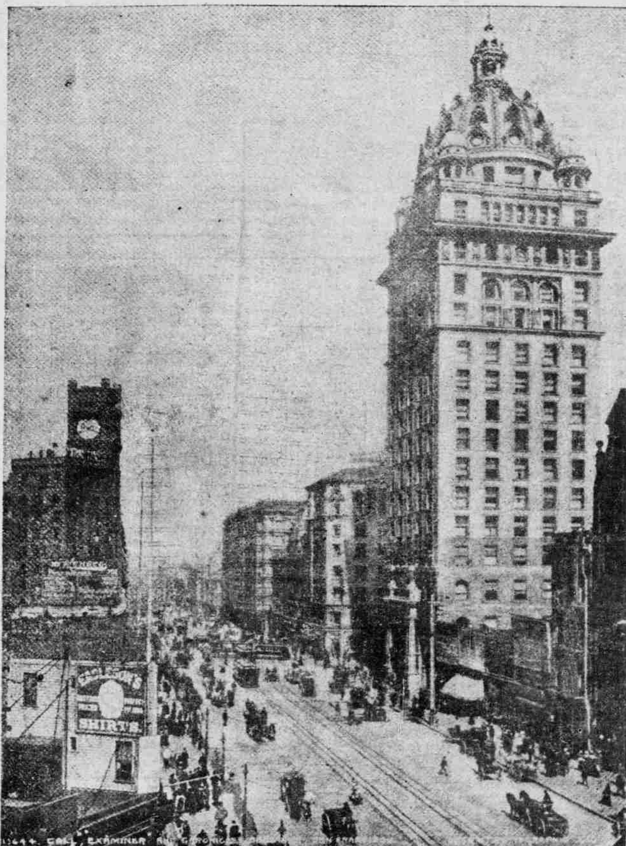
THE DESTROYED CALL BUILDING.
