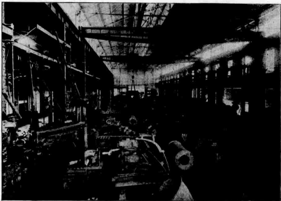
Interior View Machine Shops, Honolulu Iron Works, Showing Three Nine-Roller Mills in Process of Erection [PHOTO BY WILLIAMS, HONOLULU]
