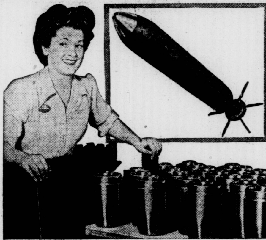
Having built more than 150,000 rockets for use on both the Pacific and European fronts, Chrysler Corporation has just been permitted by the War Department to release these photos of the projectiles. Julia Kisline, production worker at the Dodge main plant in Detroit, displays the shell noses, which are produced in quantity on machines that formerly built cars and trucks. Inset photo shows the completed rocket with fins spread as it appears in flight.
