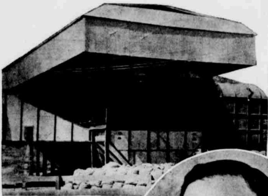
Rich potash (in bags) reclaimed through dust precipitator at a cement plant.
