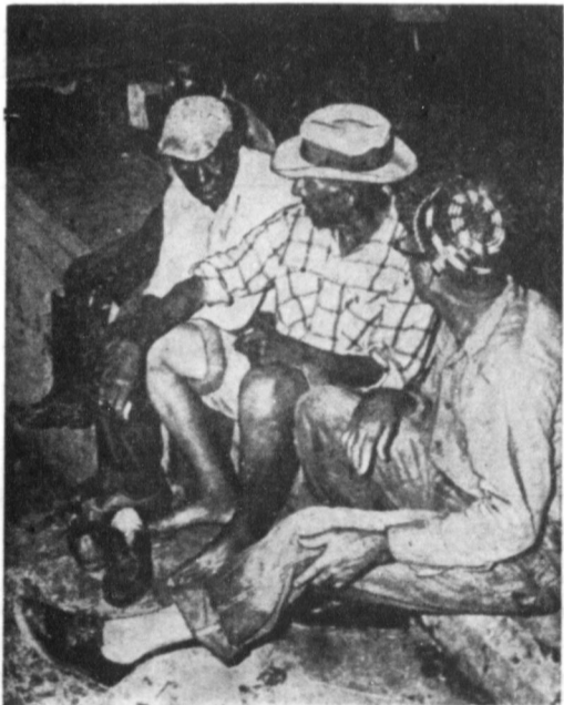
VICTIMS OF AUDREY —Driven from their homes by Hurricane Audrey, these storm victims sit outside the courthouse at Cameron, La., wondering what to do next. Their city felt the full force of Audrey's high winds and tidal waves, which destroyed almost 98 percent of the buildings. (Newspress Photo).
