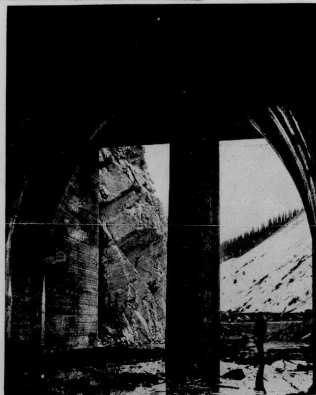
Even concrete dam construction has feature with vaulted church look. This is entrance portal to Hungry Horse dam diversion tunnel now the channel for the swift-flowing Flathead river's south fork.
