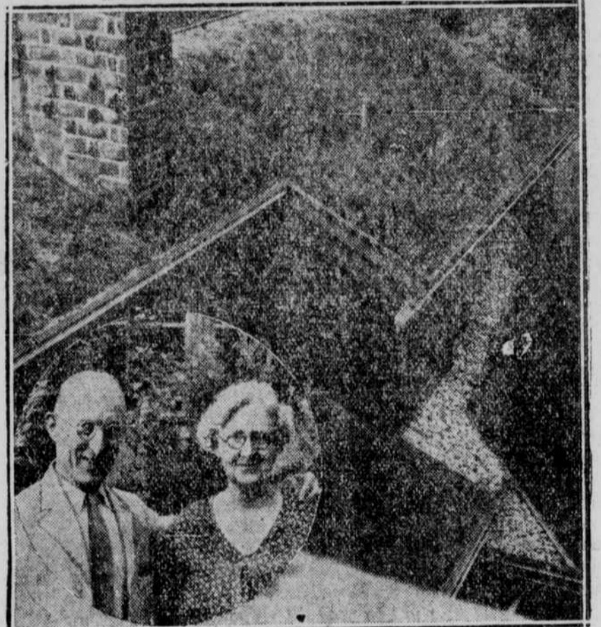
Placed on a waterproof foundation, green grass grows merrily on the roof of Louis Koefoed's home in Nassau County, L. I. Koefoed, an architect, is a specialist on roofs and has chosen the novel one shown for his own house. He claims it keeps the house warm in Winter and cool in Summer. He is shown in inset with his wife. Maybe he'll get a goat for a lawn mower.
