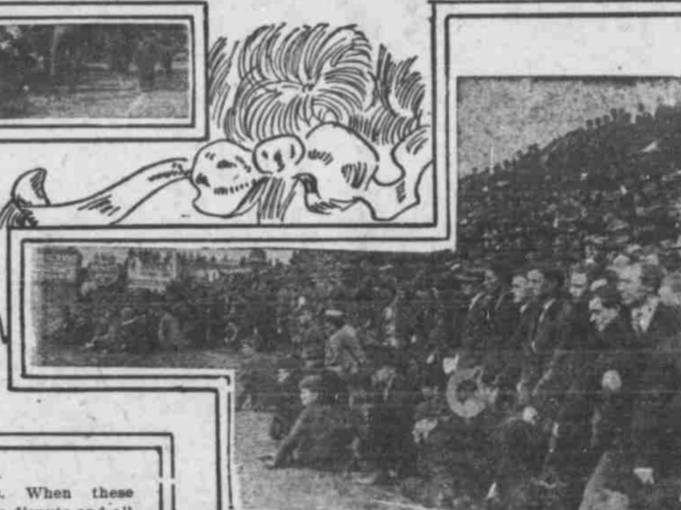
ALONG THE WEST SIDE
