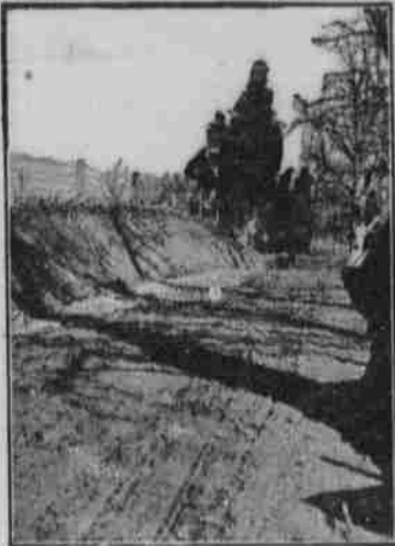
Good Road in Southwest.
