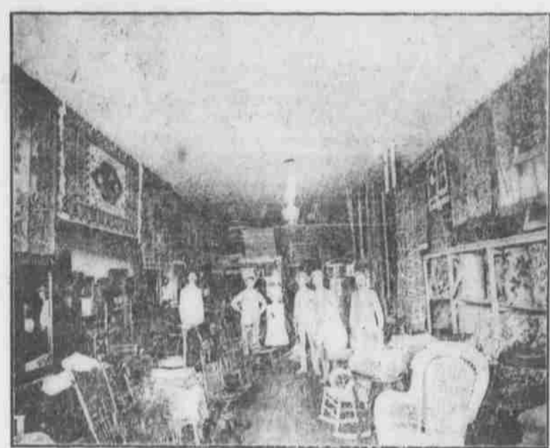
Interior View of J. A. Mahoney's Furniture Store.
