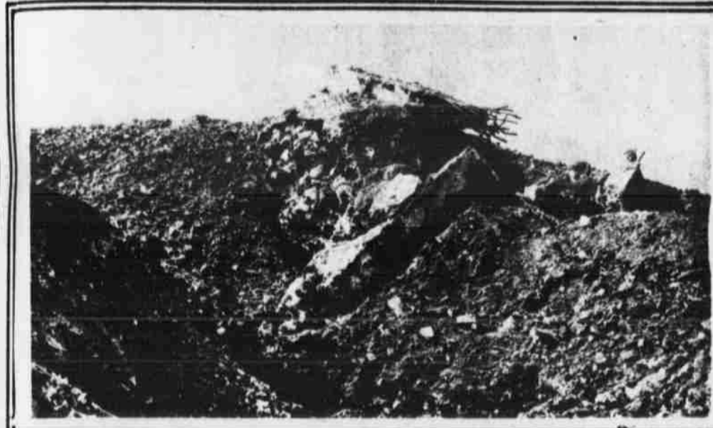
1—All that remained of one of the small forts known as points d'appui. It was built of reinforced concrete.
