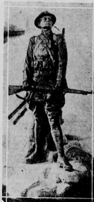
"CRUSADING FOR RIGHT" STATUE INSTALLED
