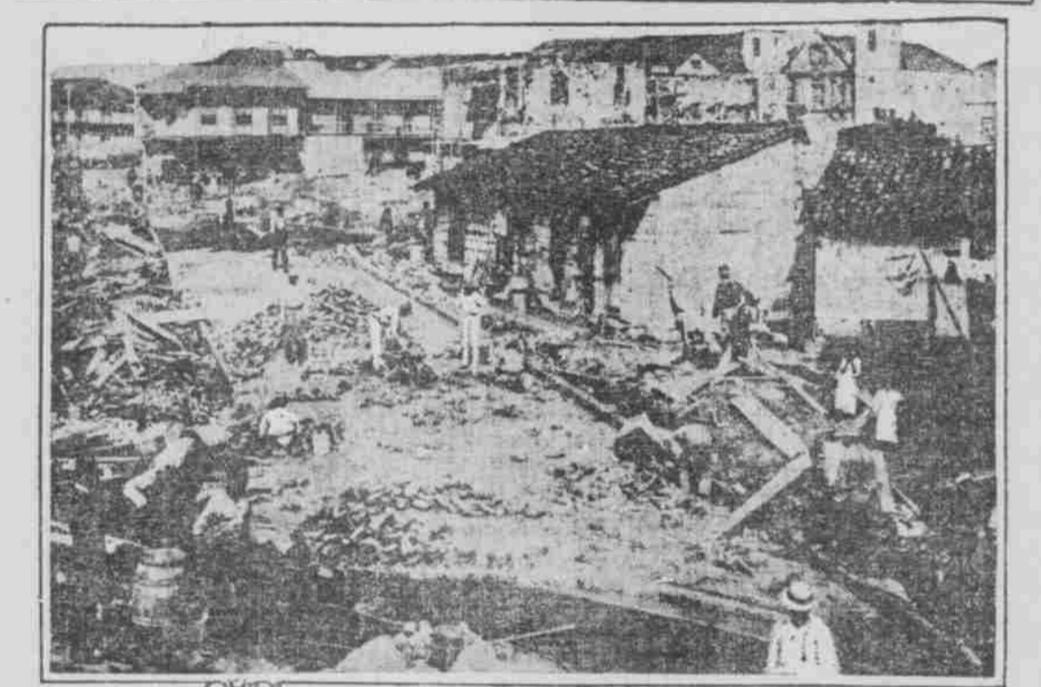
LAYING BRICK STREET IN CITY OF PANAMA.
