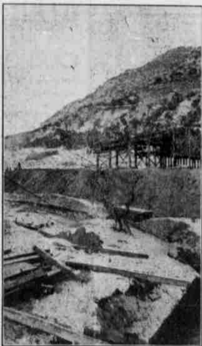
New Tipple Under Construction at Mohrland.
