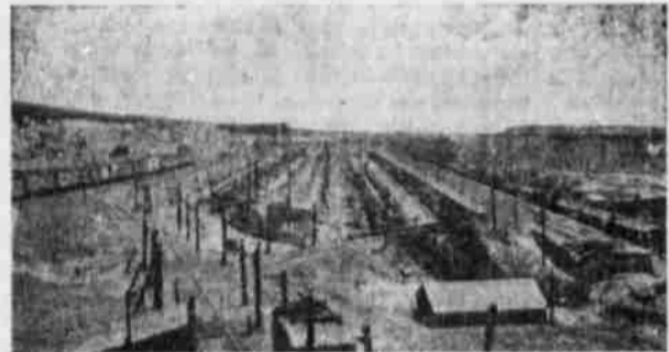
Portion of the 750 Coke Ovens at Sunnyside.
