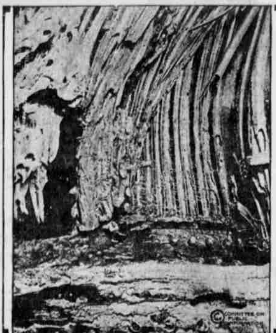
This is a graphic illustration of how the crews of the interned German ships tried to render the vessels unfit for use by the American government. The photograph shows the interior of the boiler of the Pommer, now the Rappahannock, showing how the German crew melted down the boiler by dryfiring, probably using "thermit" to intensify the heat.
